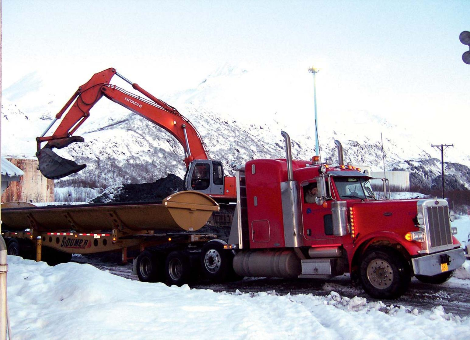
*The operator, an MLFA employee, prepares to load a Northstar Trucking Inc. side dump using an Alaska Construction Equipment Inc. 450 excavator. Approximately 40,000 tons of contaminated soil was transported from Whittier to Anchorage during the winter for thermal processing.*
