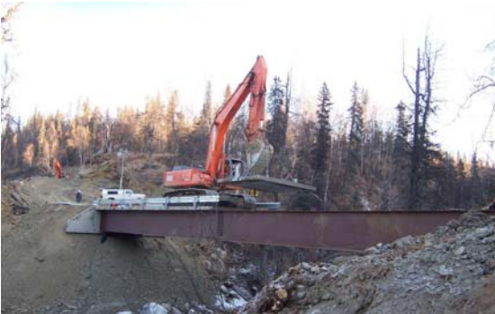
2008 Denali High Adventure Boy Scout Camp pioneer road/bridge design/build.
